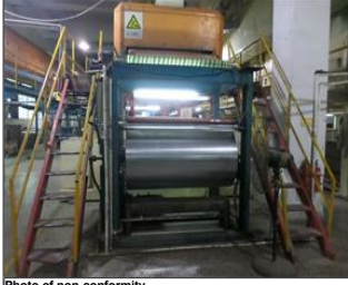
Photo of non-conformity NC3 No safety guard and warning notice.JPG
