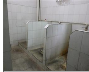
Photo of the sanitary facilities 17 toilets.JPG
