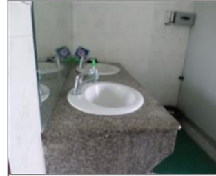
Photo of the sanitary facilities 18 The sanitary facilities.JPG
